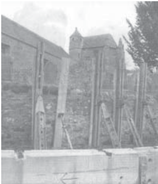
Concrete blocks protect the steel supports holding up Arbuthnott churchyard wall
